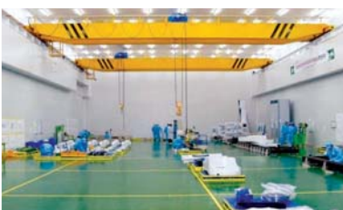
Clean Room Factory 2
